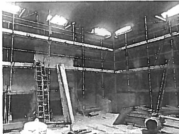
View of atrium looking towards premises
