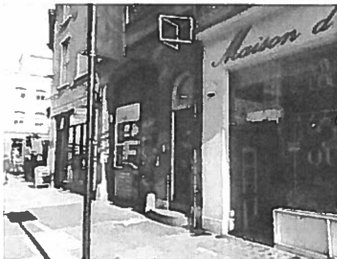
Building frontage viewed from the south
